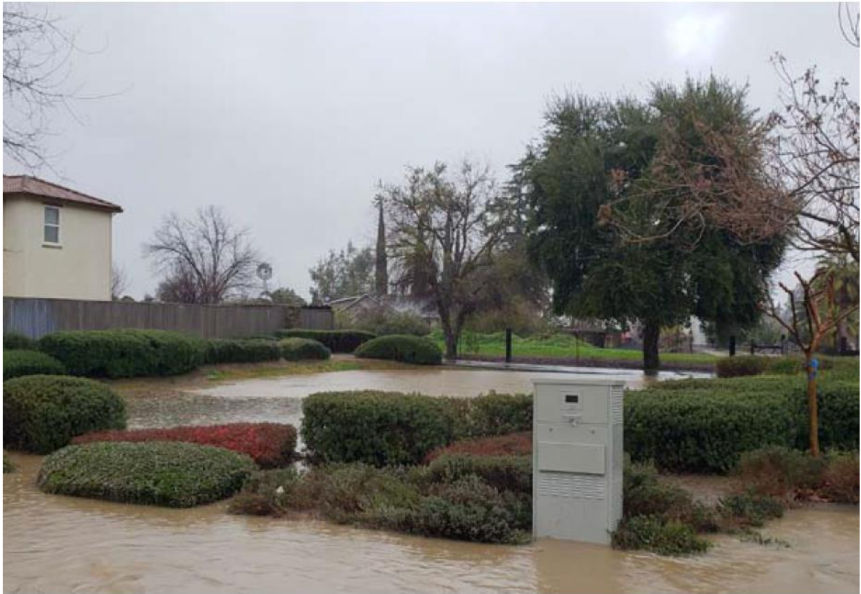
Figure D-3 CCSD – 2019 Flooding on a Flood Retention Pond at Barbara Way in River Glen Neighborhood
