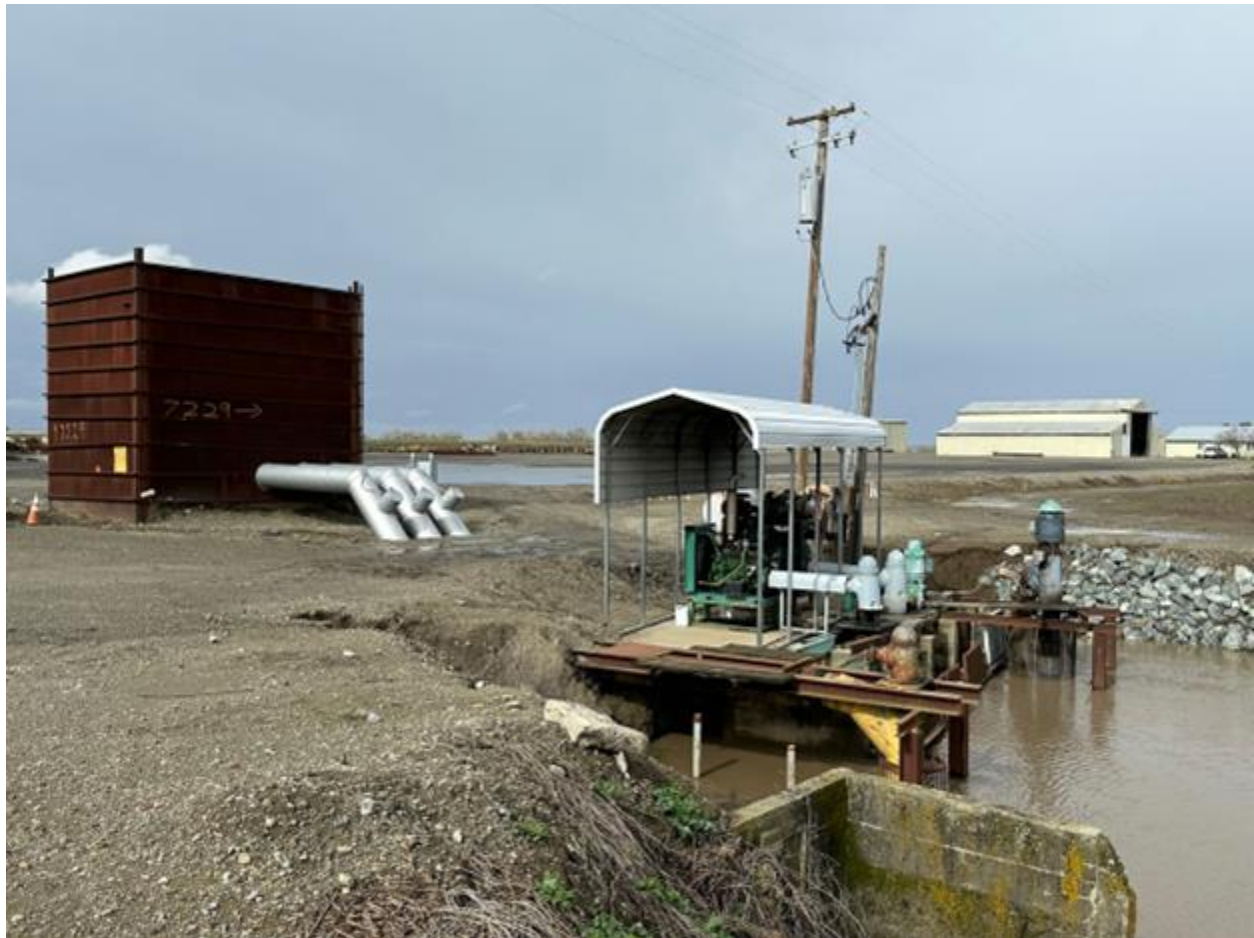
Figure G-3 RD 479 Steel Box
