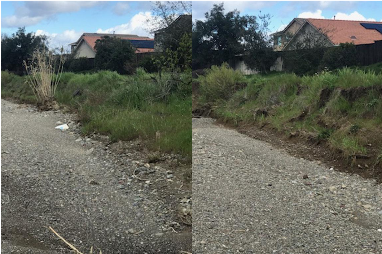
Figure D-8 CCSD – Streambank Erosion on Salt Creek
